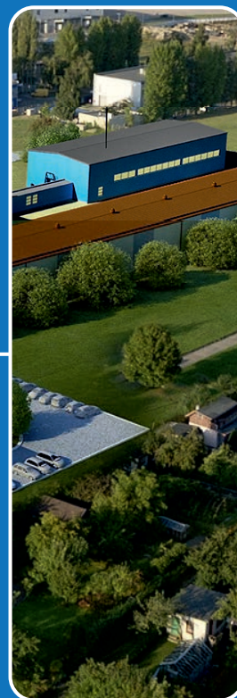
Complex of CTO facilities
